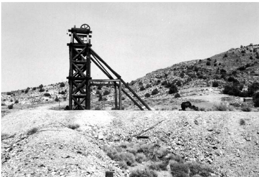
“A ‘Colorado style’ headframe, which was unusual in Nevada, was built to pull the ore up the shaft and out of the mine.” (Photograph by Lila Lindsay, used courtesy of WCRM.)
